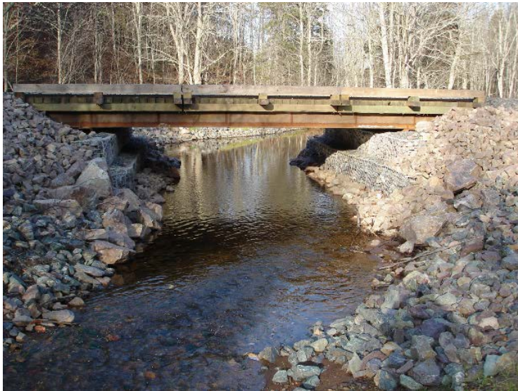
New bridge installation, Paul MacDonald, PHP
